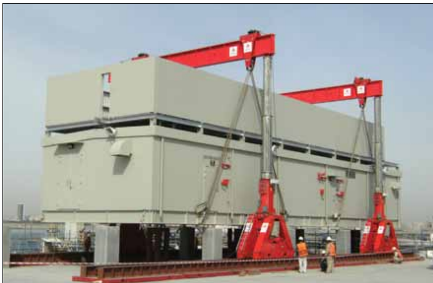
◀ SBL Series Gantry used for load out operation.
