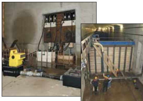
◀ Enerpac lightweight aluminum RAC-506 cylinders are ideal for wet environments such as this tunnel under the river (Holland High-Speed Train Line).
