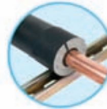
2. Pipe hanger inserts are put in place and glued to insulation.
