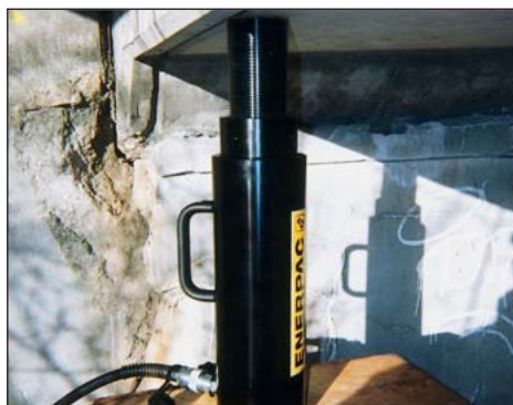
◀ The portable Lock Nut cylinder RACL-1506 used for extended load support during epoxy injection for bridge reinforcement.
