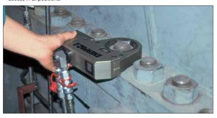
▼ An Enerpac HXD hydraulic wrench brings safety and efficiency to this flange maintenance job at a refinery.
