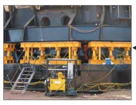
Positioning a 3500 ton dragline was successfully done with an Enerpac synchronous system. This operation provided for exact alignment of the bearing on the rail, prior to torque tightening of the slew ring bolts.
