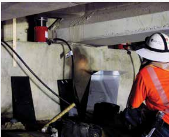
Lock Nut Cylinders lifting a bridge in Chandler, AZ
